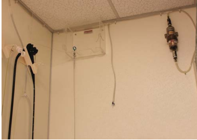
Figure 11.11 A forced-air system winds around the reprocessing room. Tubing is directed to the “clean side” of the counter for preliminary forced-air action, and at several endoscope hanger stations for an additional 15–20 min. Many endoscope hangers include areas to hang biopsy forceps for thorough drying.
